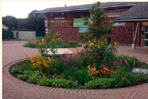
Photo: SuDS at Measham Leisure Centre
