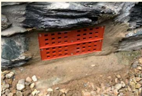
Photo: Automatically closing airbrick, Swithland
