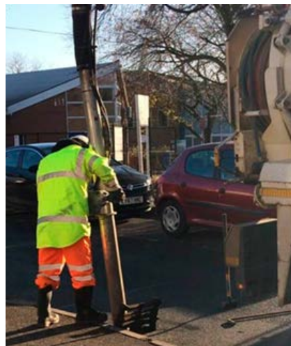
Photo: gully cleansing in Leicestershire
