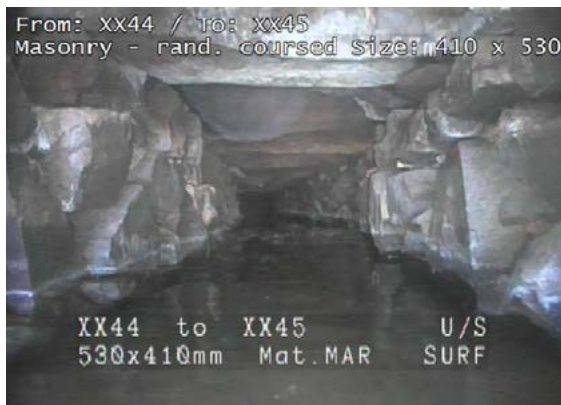
Photos: outfall (left) and CCTV survey (right)
